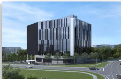
Infinaxis Data Centre, Cyberjaya
