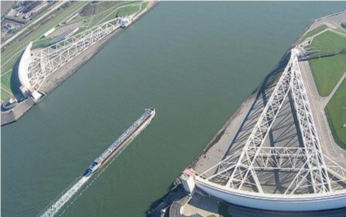
Storm Surge Barrier
