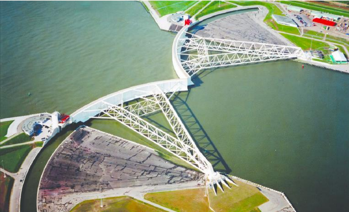
Storm Surge Barrier
