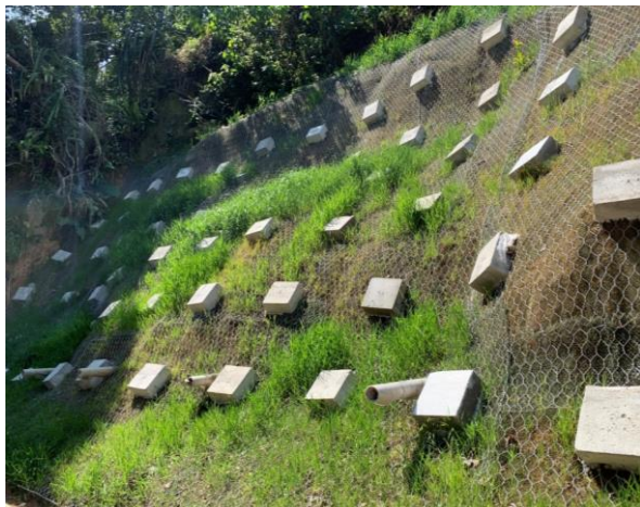
Soil-Nail tanpa Shotcrete
