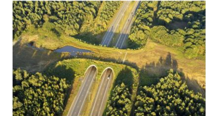
06 T1S3P1 – Viaduct Sg. Mangga
