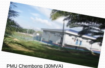
PMU Chembong (30MVA)
