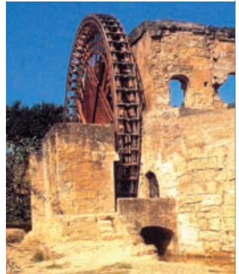
Figure 10: The water-wheel that lifted water from the Guadalquivir into the gardens and the houses of Cordoba.
