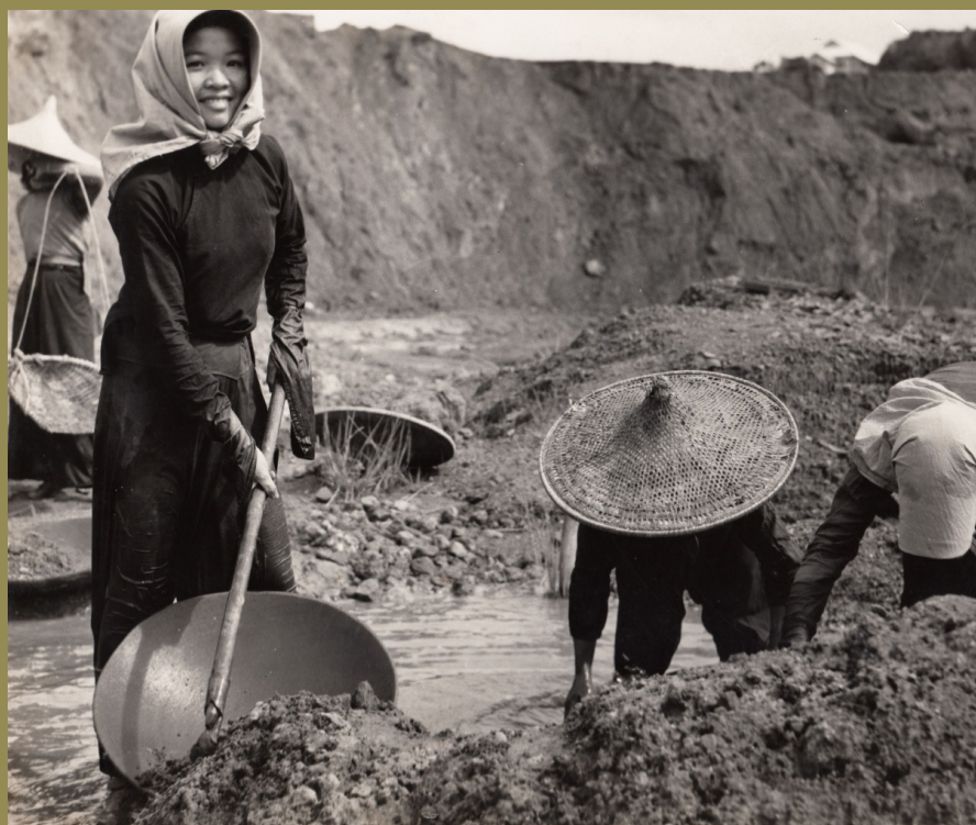
Mining tin ore by panning
